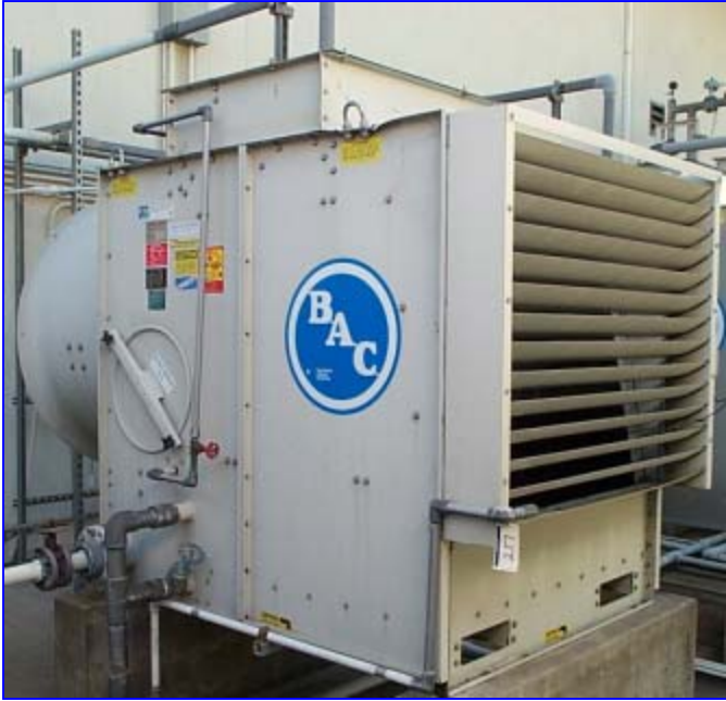
Baltimore Water Cooling Tower, Model FXT-26R S/N U12879601MAD, (CTI 92-11-01), with Marathon 3 hp pumps.
