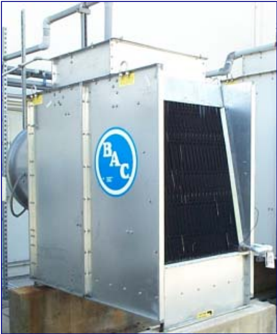
Baltimore Water Cooling Tower, Model FXT-16, S/N U025573801MAD, (CTI 92-11-01), with Marathon 1.5 hp pump.
