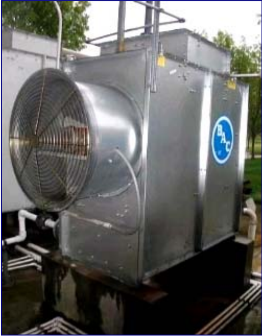
Baltimore Water Cooling Tower, Model FXT-16, S/N U025573801MAD, (CTI 92-11-01), with Marathon 1.5 hp pump.
